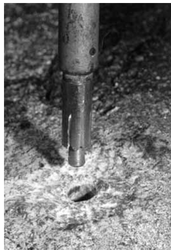
Wedge in, bolt ready to set
