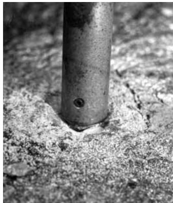
Drill until the anchor is 2 mm to 3 mm below the surface
