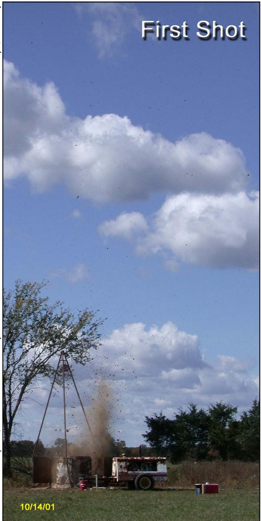
using an 8-hole pattern that adds 2 holes nearer to the 9-inch pilot hole. The 8-hole pattern is the currently preferred pattern. When the 8-hole pattern is used the 2 holes near the pilot hole are loaded with zero delay detonators. Two of the neighboring outer holes have an intermediate delay and the remaining four charges go off last. The first explosion opens a hole for the next blast that in turn opens a hole for the material from the final blast.
